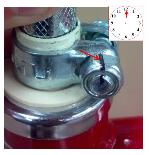
With the nut and bolt surfaces in alignment, draw a line on the top surface of the nut at the 12 o'clock position.
